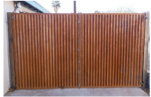
Corrugated Steel Vehicle Gate
