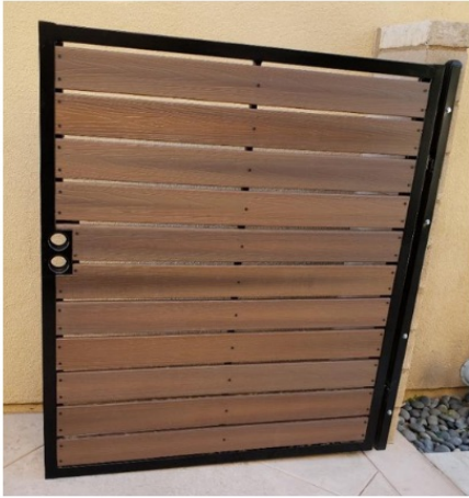
Steel Frame & Wood Gate
